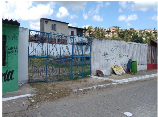
Figure 5: Elevator Station- Caetes III
