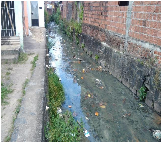
Figure 7: Sewage ditch – Centro
