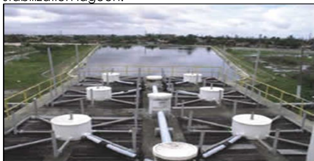
Figure 1 - Mangueira WWTP UASB Reactor and stabilization lagoon.
