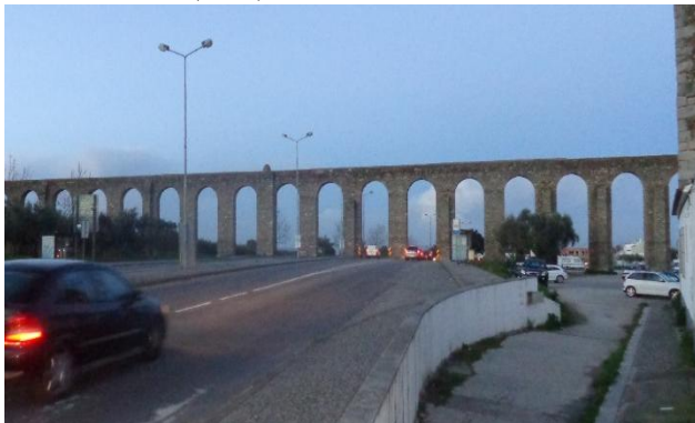
Figure 2 – Roman Aqueduct Água da Prata – Évora. Source: Author (2013).
