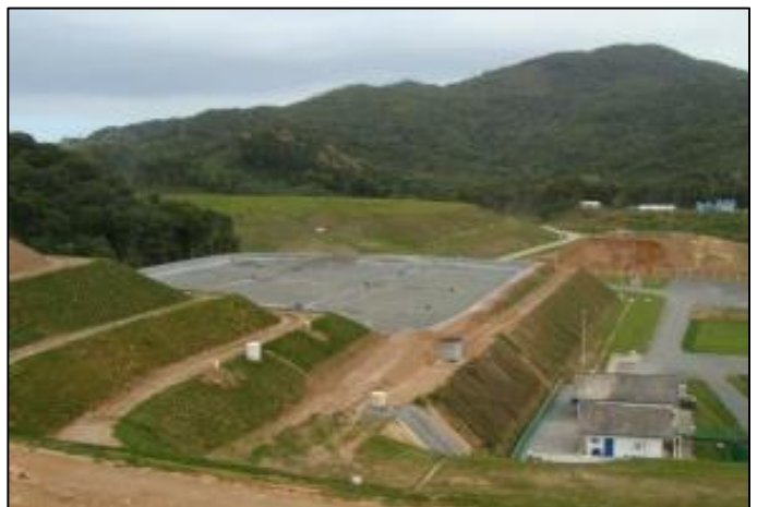
Figure 02. Landfill in ditches. Source: Machado, 2013
